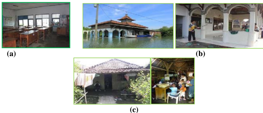
Fig.3 Condition of Facilities in Bedono Village Source: Field Observation, 2014
